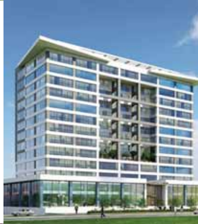
CAPITAL TOWER / İSTANBUL
